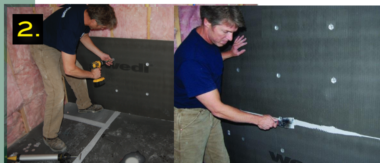
Attach Wallboard and Seal Joints
