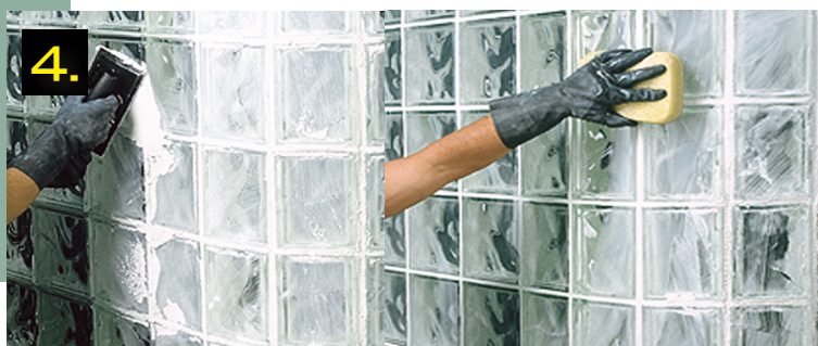
Grout All Joints Between Glass Block
