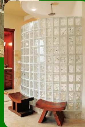
Soft Radius 6 x 8 Straight Block with Tapered Joints
