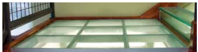
Total time for this stair landing: approximately 2 hours.
