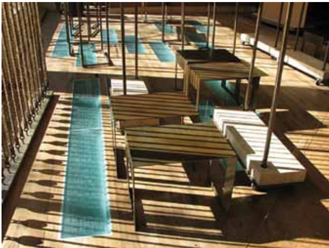
These GlassWalk SG inserts were sized to fit between existing floor joists, adding a distinctive element to a retail decor . . .
